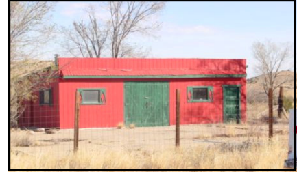
Workshop—wired w/wood stove
